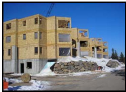
Construction continues at Touchmark despite the harsh weather.
